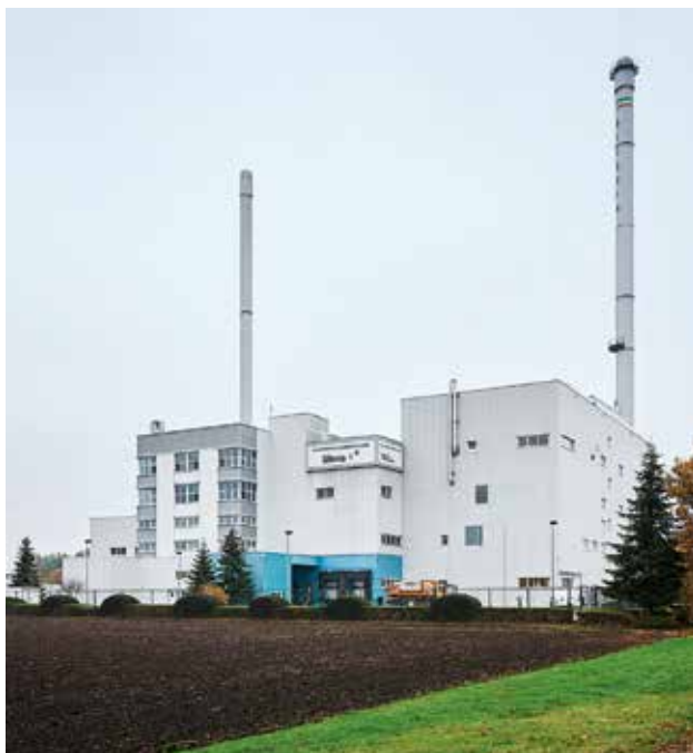
Silesia plant in Kalkar: the focus is on the production of flavor powders for the food industry.
